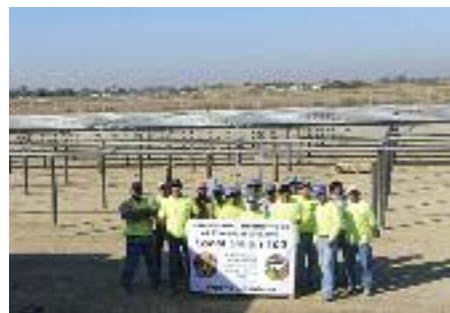
IBEW Fresno, CA, Local 100 crew installs VF Outdoor Inc. solar project.
