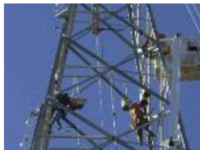
IBEW Springfield, IL, Local 51 members at work on the Havana 138-kv rebuild.
