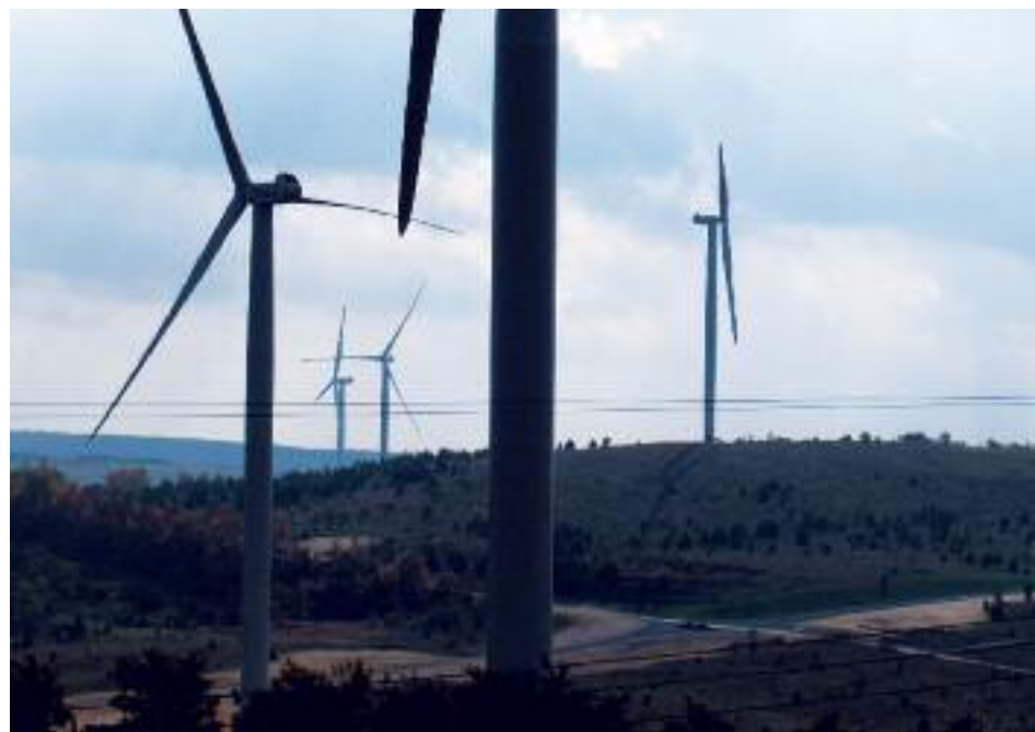
Members of Philadelphia Local 126 connected 10 miles of cable between windmills in rural Somerset County.
