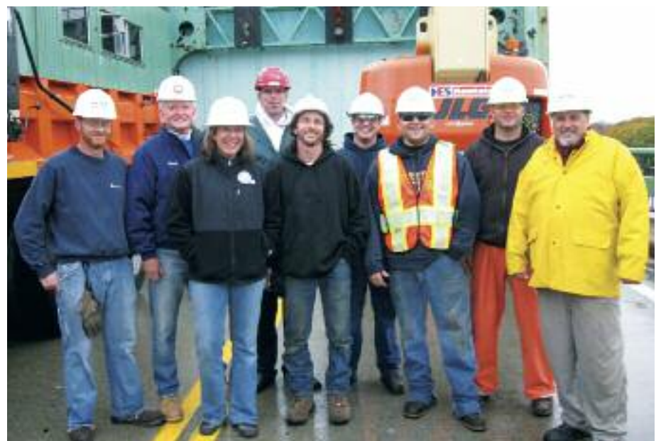
Members of Dover, N.H., Local 490 repaired the failed draw on the Sara Long Memorial Bridge. The bridge, a critical link between New Hampshire and Maine, was completed in 3½ months by 12 members of the local. Yates Electric employee Brian Skeffington, at left, with Second District Vice President Frank Carroll, International Office employee Tina Thoman, Local 490 Business Manager Scott Ricard and Yates Electric employees Jeff Brousseau, James Paradis, Keith Kearney and project foreman Tom McLaughlin.
