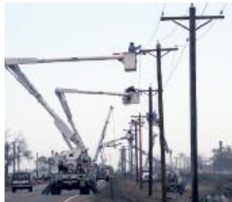
IBEW Local 667 members restore power to the town of Ordway, CO.
