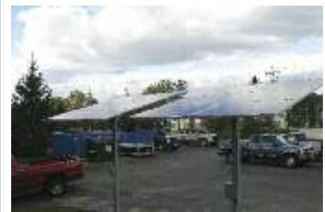
Local 86 JATC Training Facility solar array installation.
