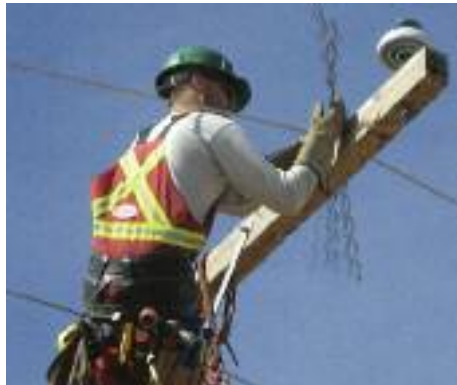
Local 254 power line apprentice Steve Quinlan competes at lineman's rodeo.
