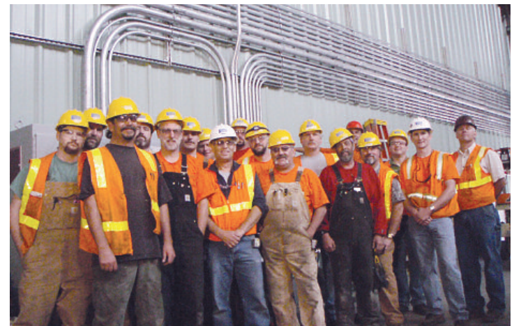
Local 280 members at work at the Freres Plywood Cogeneration plant.
