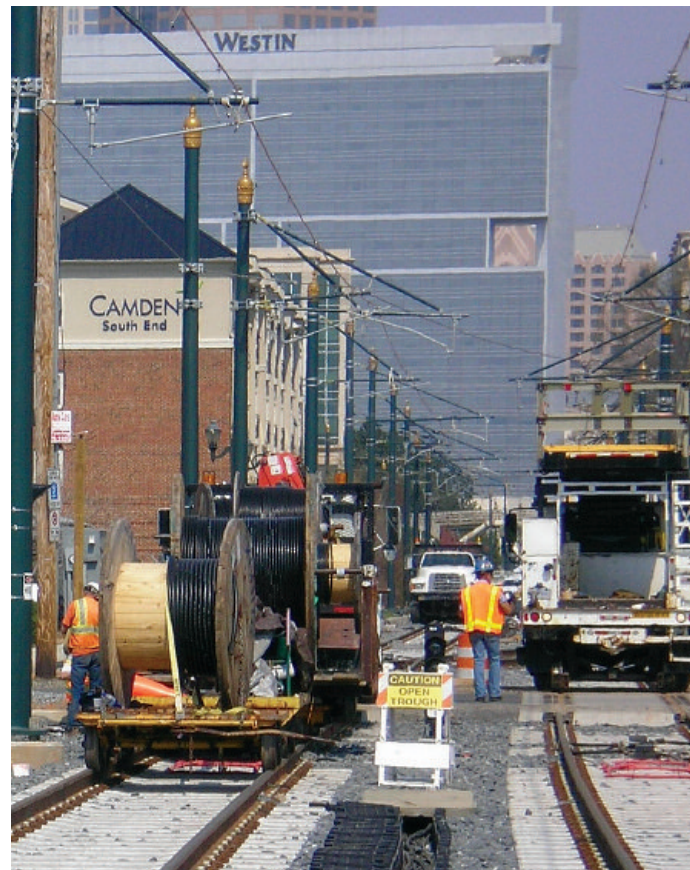
Charlotte, N.C., Local 379 members wire the first light-rail system in North Carolina.
