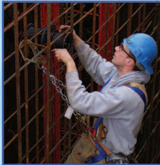
Journeyman wireman Michael Laidman
