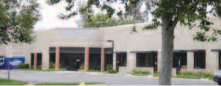
Local 47's new office purchased for its Outside Construction Unit. The 6,300 square-foot facility provides plenty of room for offices, dispatch and meetings.
