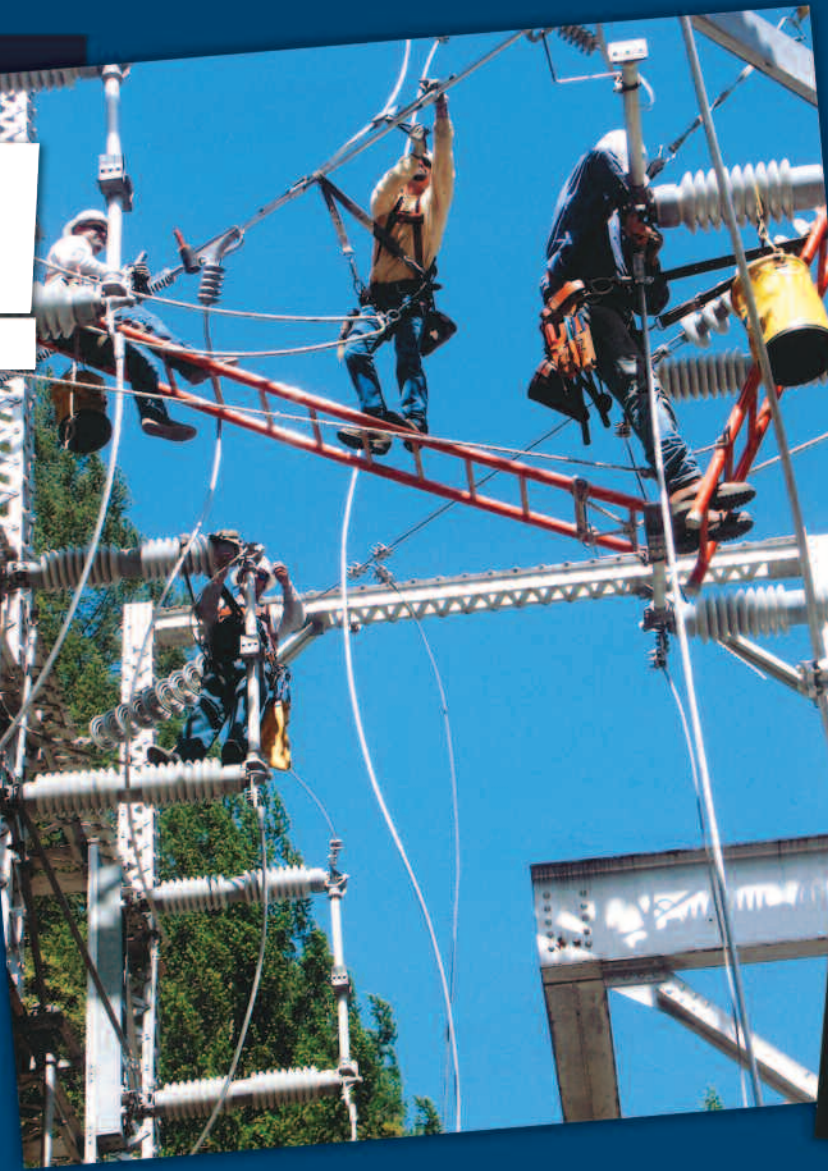
Second Place Winner Michael D. McCarty, Vacaville, California, Local 1245. A substation maintenance electrician at Pacific Gas and Electric's El Dorado power house, McCarty said, "I saw lineman from PG&E's grid maintenance and construction department replacing conductors and was impressed with how they were set up on the job with ladders and safety gear."
