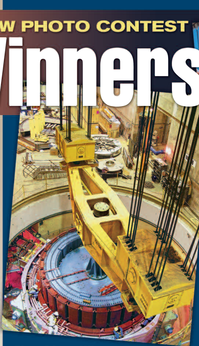
First Place Winner Ron Grant, Los Angeles Local 18. L.A. Department of Water and Power electrical repair shop employees re-install Castaic Power Plant's Unit 6 generator rotor. Overhead cranes are joined to support the weight of the 550-ton rotor. The union members are guiding the rotor into place after hanging padded spacers against the stator.
