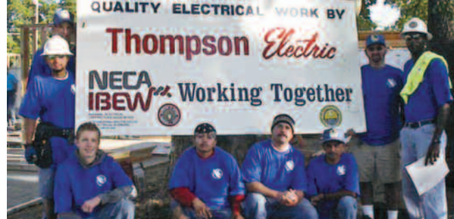
In Sacramento Local 340 employers and volunteer electricians wired a Habitat for Humanity home on Labor Day weekend.
