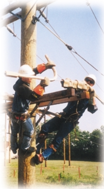
Trainees learn the lineman's craft on the ALBAT training grounds.
