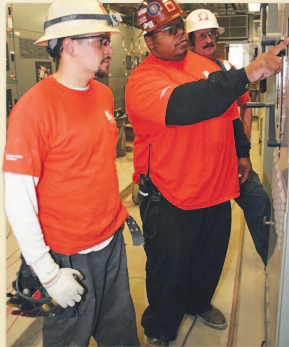
John Harriel Jr. plans job with apprentice Alex Suarez, left, and journeyman wireman Larry Wernli.
