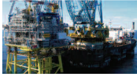
The heavy lift vessel Saipem 7000 places the new compression deck platform on the jacket for installation by IBEW Local 625 members working in the offshore Nova Scotia gas industry.
